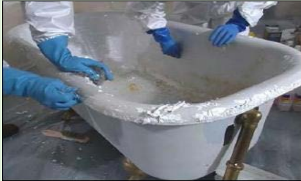
Removing paint & coatings with methylene chloride-based stripper
