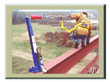
Remember - The anchorage point for fall arrest systems must be capable of supporting **5000 lb.** for each worker or used as part of a complete PFAS which maintains a safety factor of at least two and under the supervision of a qualified person.
