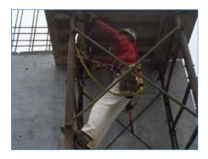
Full body harnesses are often designed with D-rings on each side of the waist belt so that the harness can be used both as a PFAS and as a positioning device.
