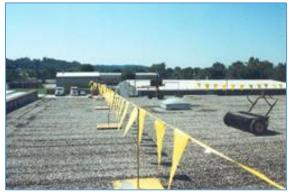
The warning line must have a **strength of 500 lbs.** It must have **high visibility flags every 6 feet.** The lowest point of the line must be between 34 and 39 inches above the roof surface.
