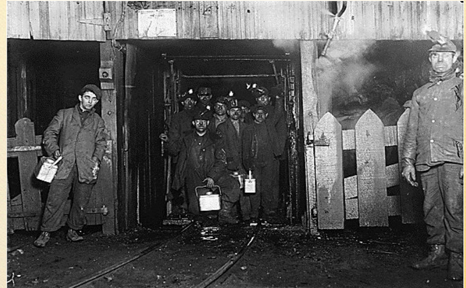
Miners waiting for the cage to go up at the end of the day. Two sides of the cage are open; the other two sides have little protection. The cage is usually crowded. S. Pittson, PA 1
