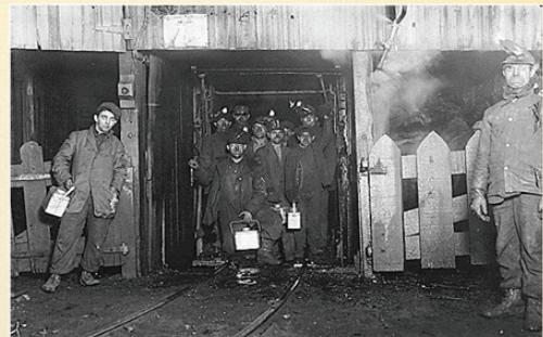
Miners waiting for the cage to go up at the end of the day. Two sides of the cage are open; the other two sides have little protection. The cage is usually crowded. S. Pittson, PA 1
